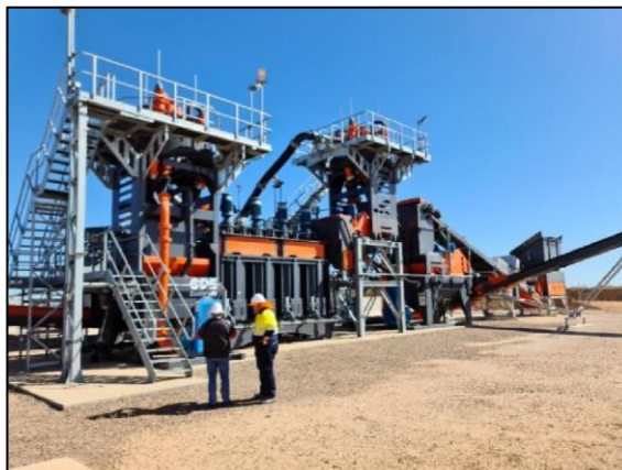
Figure 2 – Completed Trial Processing Plant (240ktpa) at the Ardmore Phosphate Project
